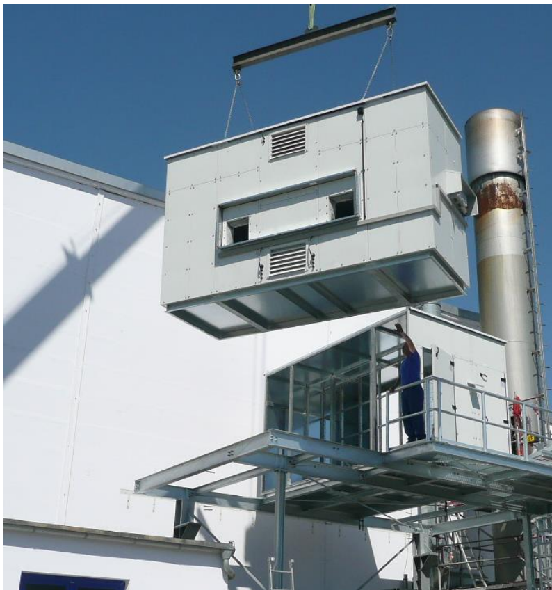
Installation of the exhaust air system
