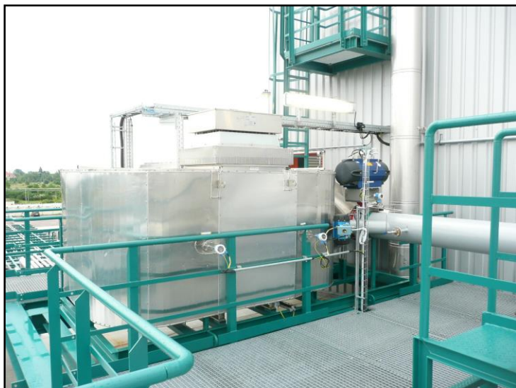
Catalytic oxidizer (CATOX)
