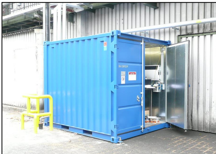
Non-catalytic reduction (SNCR), installed in ISO-Container; stack with dosing platform
