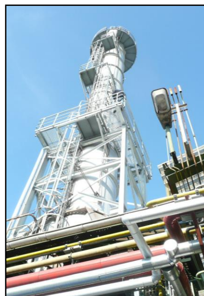
Non-catalytic reduction (SNCR), installed in ISO-Container; stack with dosing platform
