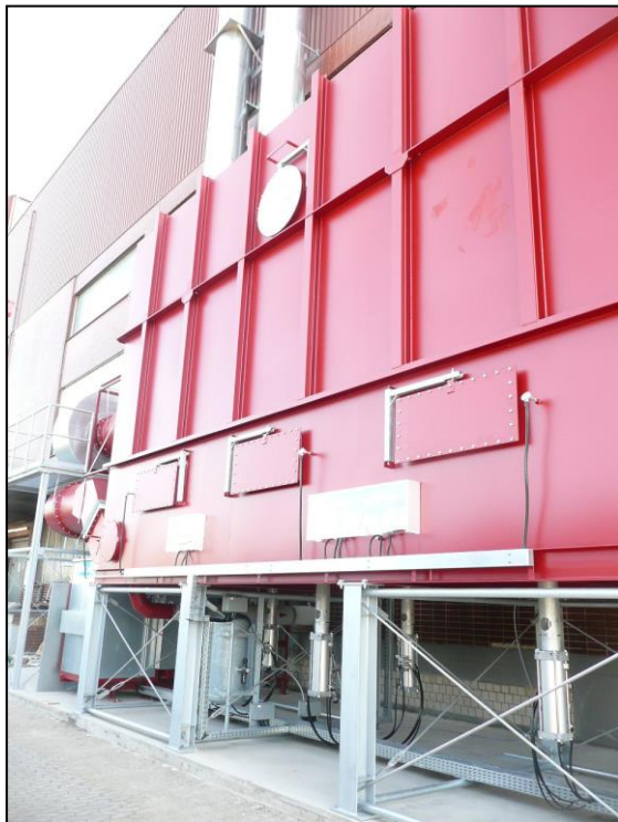
RNV- 3 chamber unit with ceramic storage mass
