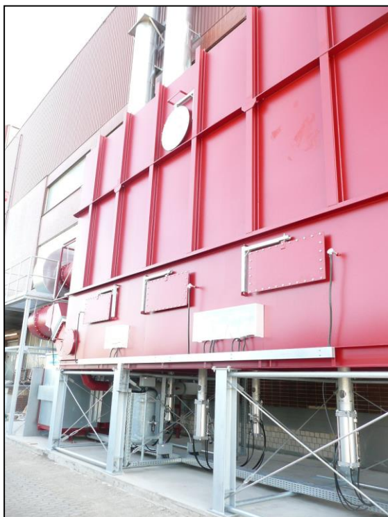
RNV- 3 chamber unit with ceramic storage mass
