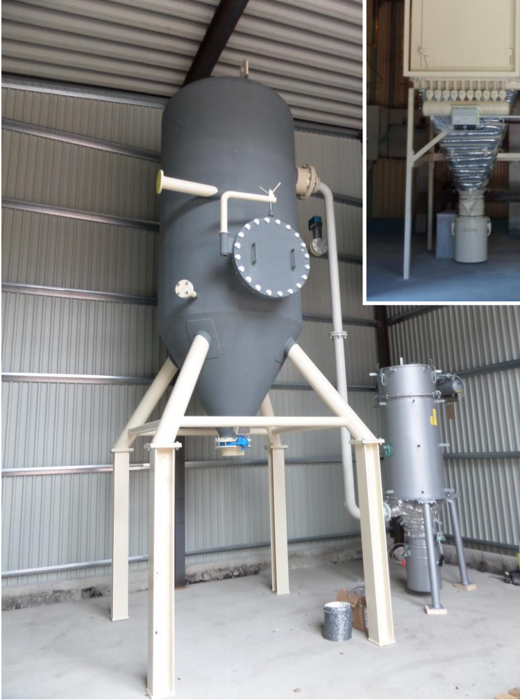
Equalizing vessel and round dust filter
